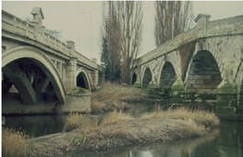
Bridges at Atcham
